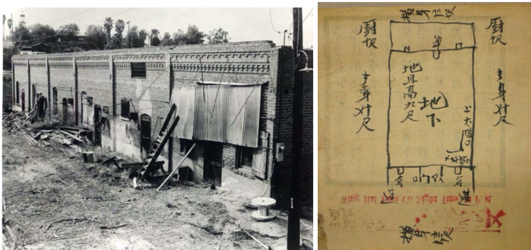
Figure 7.3. Left, front of the western brick building with an additional sixth bay, 1959. Courtesy of the Save Our Chinatown Committee. Right, layout sketch of sixth bay added some time after 1908. From the Wong Sai Chee records held at the Museum of Riverside.
