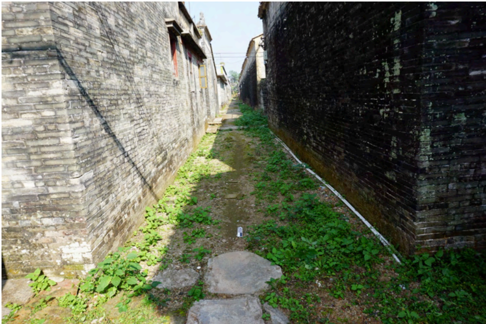
Figure 5.7. Conditions in Zone C north-south alley NS 2B, facing north.
