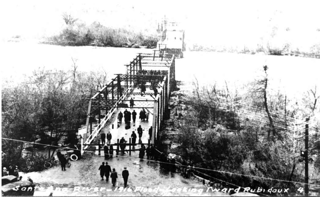
Figure 4.8. Photo of the washed-out bridge between Riverside and West Riverside after the 1916 flood. Courtesy of Nancy Wey Papers, UC Berkeley Ethnic Studies Library.
