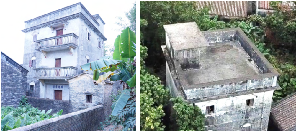
Figure 8.8. The eastern side (left) and flat reinforced concrete roof (right) of Wong Shoon Jung's three-story house built in the late 1920s or 1930s.
