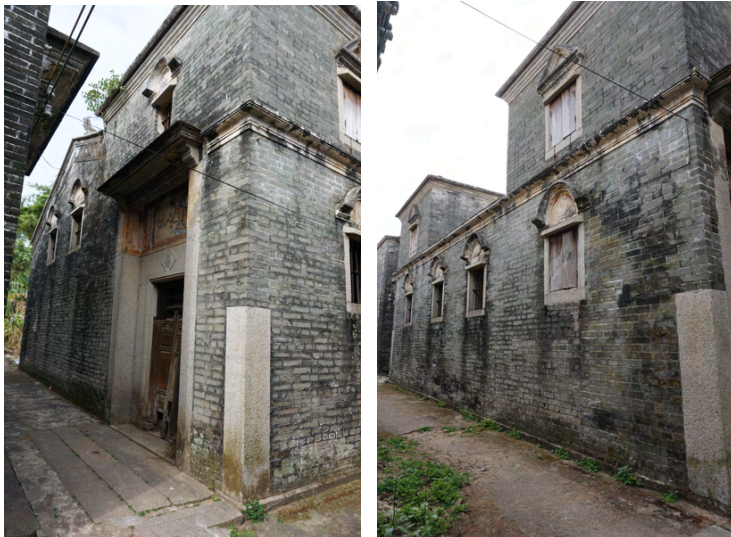
Figure 8.10. North side (left) and east side (right) of Wong Chun San's home built in the 1930s.
